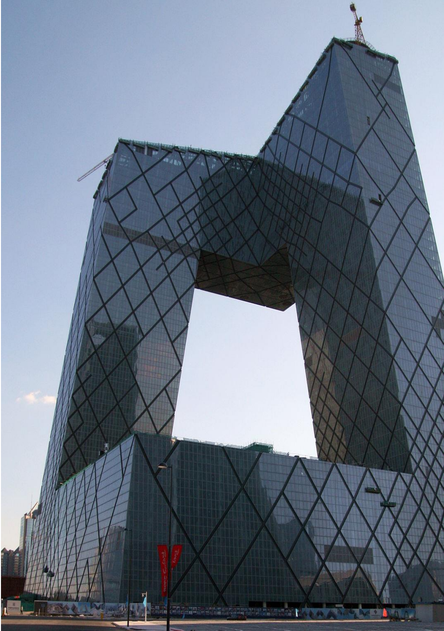
Gambar 3.11 Detail Eksterior CCTV . [ https://en.wikipedia.org , akses 21 Desember 2018]
