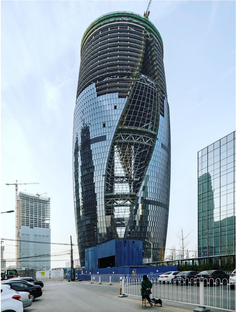
Gambar 3.30 Progres Konstruksi Leeza Soho Tower . [ https://deskgram.net , akses 28 Desember 2018]
