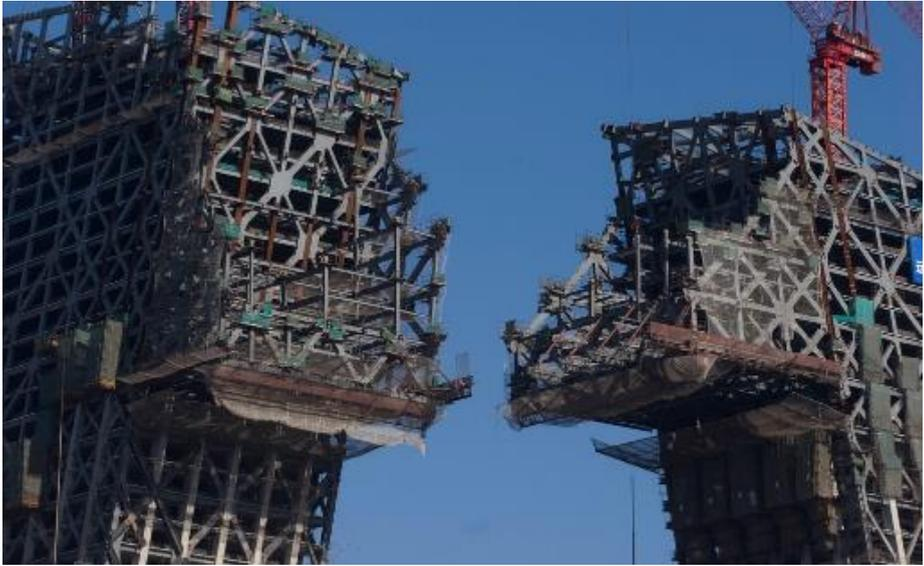
**Gambar 4.29** Detail Konstruksi CCTV [<https://www.flickr.com>, akses 22 Desember 2018]
