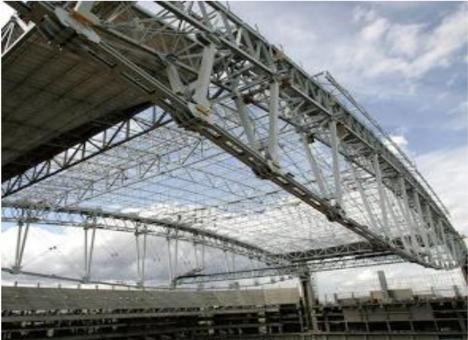
**Gambar 5.39** Detail Struktur Atap *University of Phoenix Stadium*.
