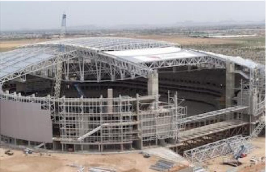
**Gambar 5.37** Progres Konstruksi *University of Phoenix Stadium*.
