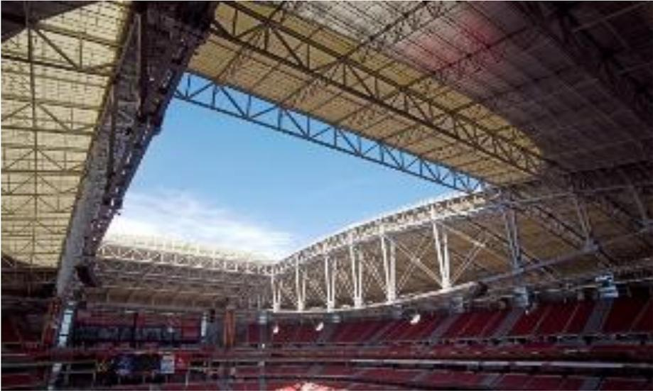
**Gambar 5.41** Detail Struktur Atap *University of Phoenix Stadium*.
