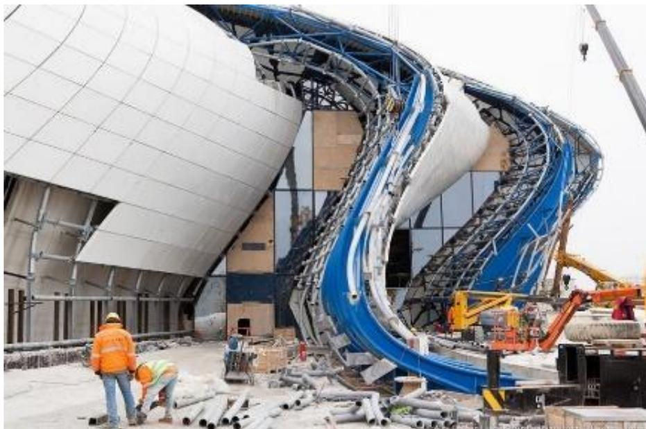
**Gambar 6.36** Detail Konstruksi *Heydar Aliyev Center* [<https://www.inexhibit.com>, akses 27 Desember 2018]
