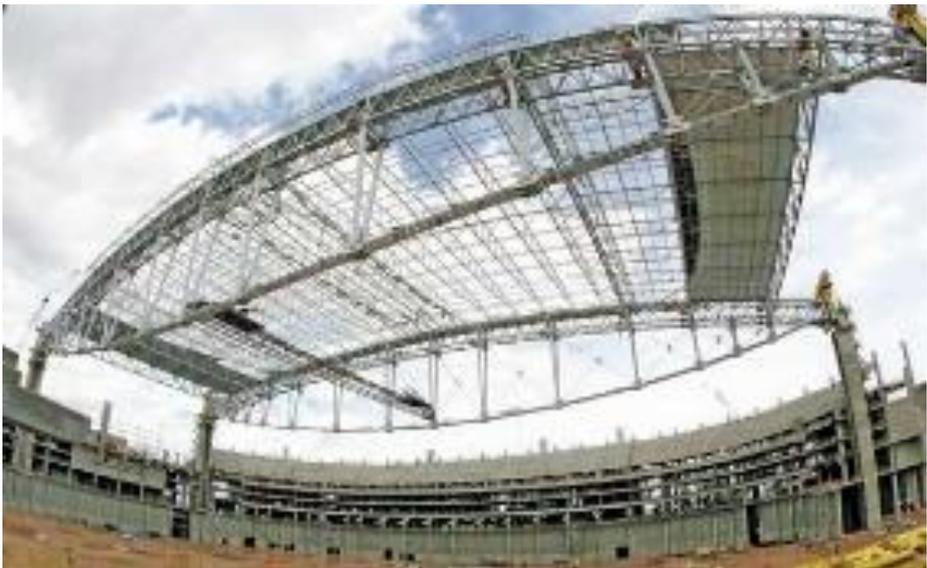
**Gambar 5.40** Detail Struktur Atap *University of Phoenix Stadium*.
