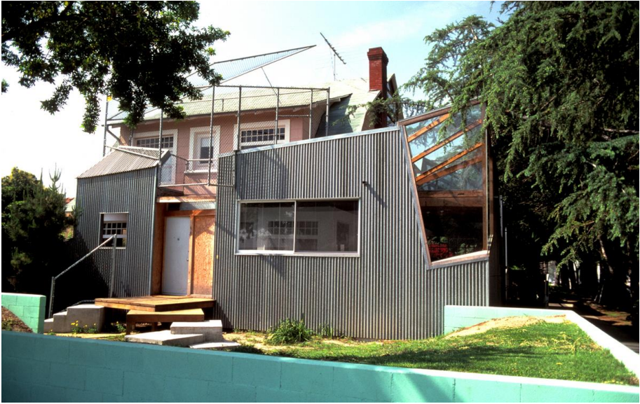
Gambar 4.26 Gehry House , Santa Monica, California (1978) karya Gehry ( http://www.usmodernist.org , akses 15 Desember 2018)
