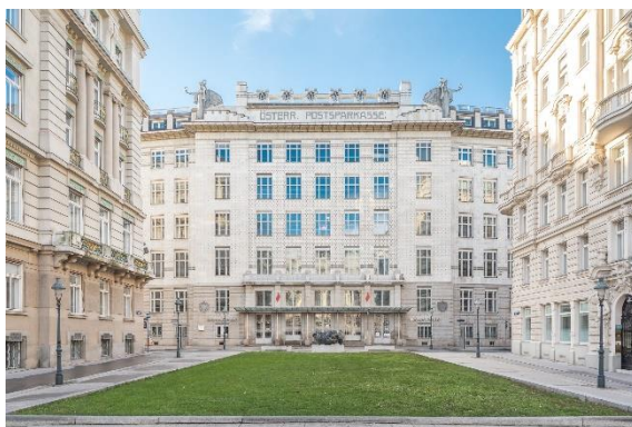
Gambar 3.52 The Austrian Postal Savings Bank , karya Wagner (1904) ( https://divisare.com , akses 30 Maret 2020).
