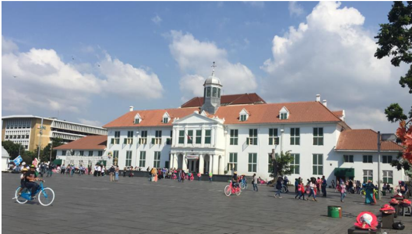
Fig. 1. The Museum Fatahillah under renovation (Purwantiasning, 2015).
