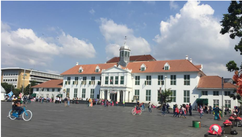
Fig. 1. The Museum Fatahillah under renovation (Purwantiasning, 2015).
