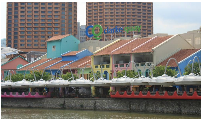
Fig. 4: Colourful buildings within area of Clarke Quay Source: Private Documentation, 2013
