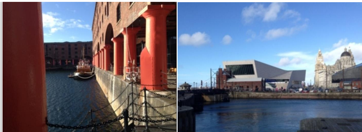
Fig. 8a, 8b: Today's pictures of old Albert Dock, left picture shows the view of Albert Dock which still remains the same character of red bricks and red pillars, this row of building consist Tate Gallery, Museum of Maritime, Cafes, Restaurants and Bars. And the right picture shows the face of another side of Albert Dock area which consist new modern building – Museum of Liverpool which contextual with the character of waterfront area.
