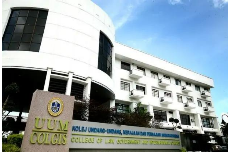
Gambar 4.1.5 Tampak Depan School of Government University Utara Malaysia Sumber: Observasi (2023)
