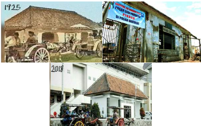
Fig. 11a, 11b and 11c. Pasar Legi Parakan is one of historical building in Parakan since colonial era in 1925 and it has been demolished and relocated in new place in 2014 and has been finished the construction in 2017
