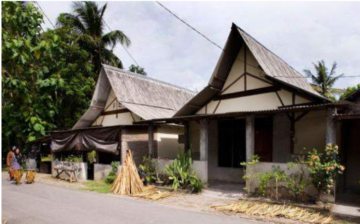
Gambar 2: Bentuk atap Rumah Ngibikan pasca gempa Sumber: Recontruction of Ngibikan Village, Brigitte Shim, 2008
