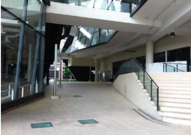
Figure 11 and 12: those figures show the area of pedestrian within campus area of Lassale. This pedestrian area is heading to enter inside the campus area. The using of material on the floor giving a comfortable feeling for the users. Some parts of the floors have been designed by putting some glasses to give natural light for basement floor.
