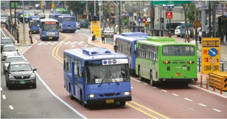
Figure 5. A Seoul BRT station with overtaking lanes. Source: Seoul Metropolitan Government [17].
