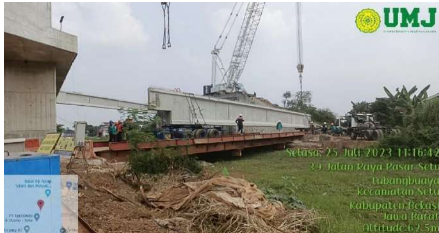
Gambar 4.1 PCI Girder
