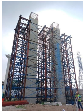
Gambar 4. 30 Shoring pier head
