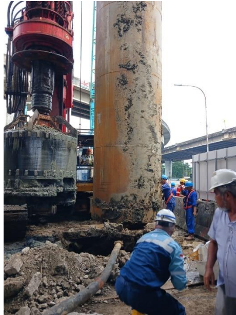
Gambar 4. 7 Instalasi temporary casing
