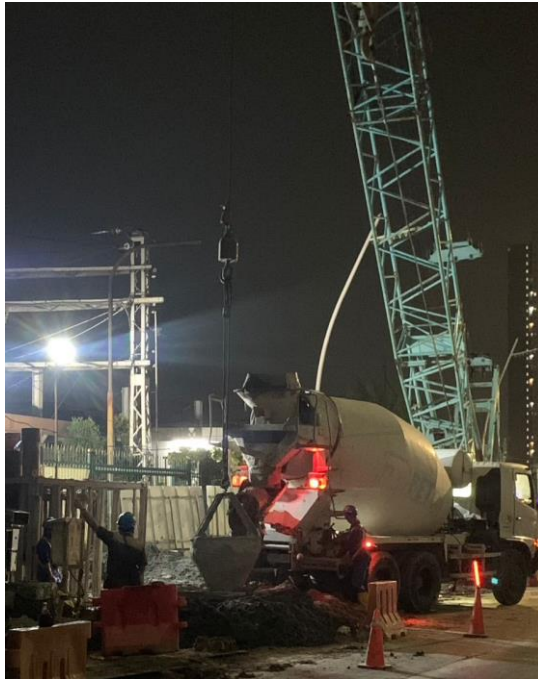
Gambar 4. 14 Pengecoran bored pile
