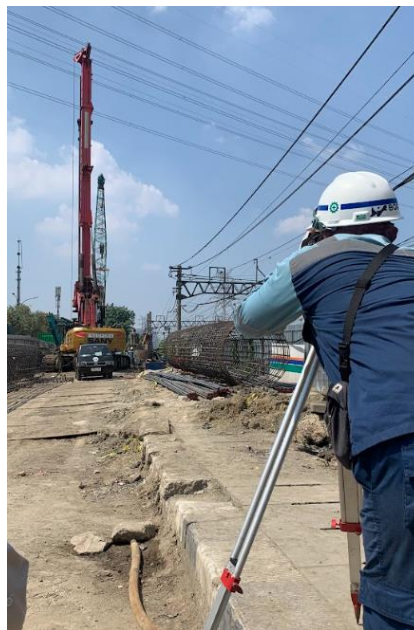
Gambar 4. 5 Staking out
