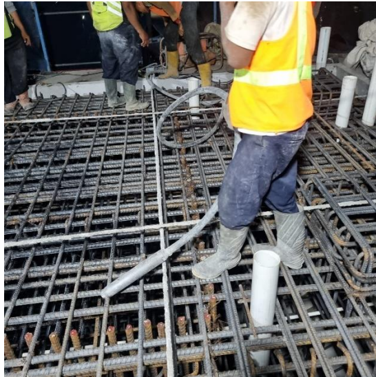
Gambar 4. 32 Pengecoran pier head
