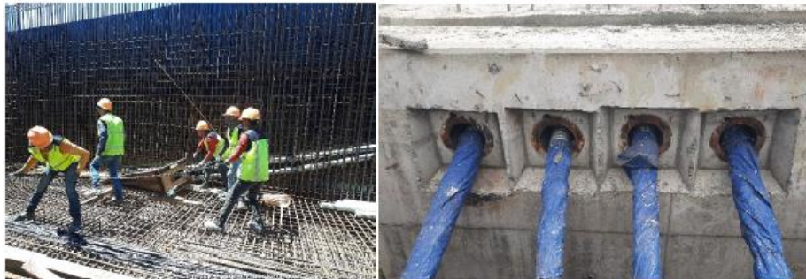
Gambar 4. 36 Proses instalasi strand
