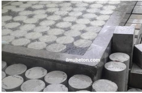
Gambar 2.10 Proses curing beton
