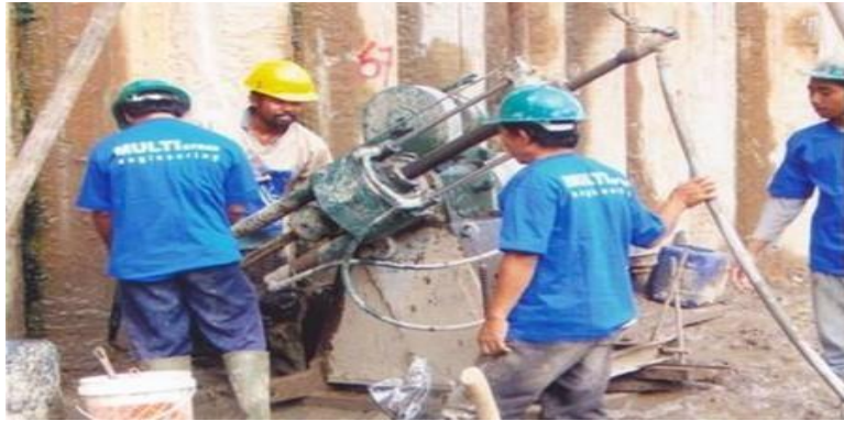
Gambar 4. 22 Proses Bore Pile wall casting work
