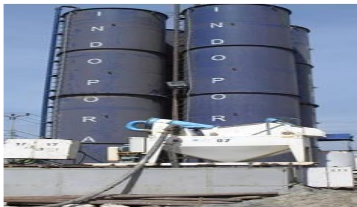
Gambar 4. 33 Silo Bentonite
