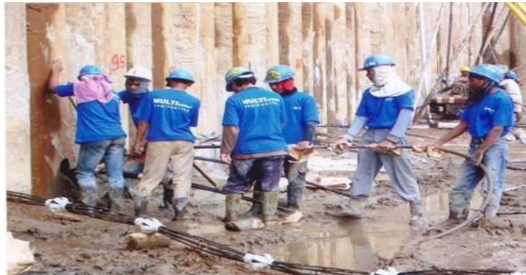
Gambar 4. 25 Proses Grouting Ground Anchor
