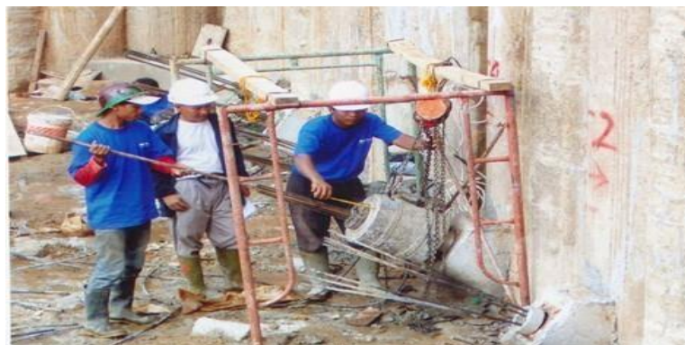
Gambar 4. 26 Proses Stressing Ground Anchor
