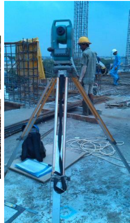
Gambar 4.37. Pekerjaan Penentuan AS Kolom
