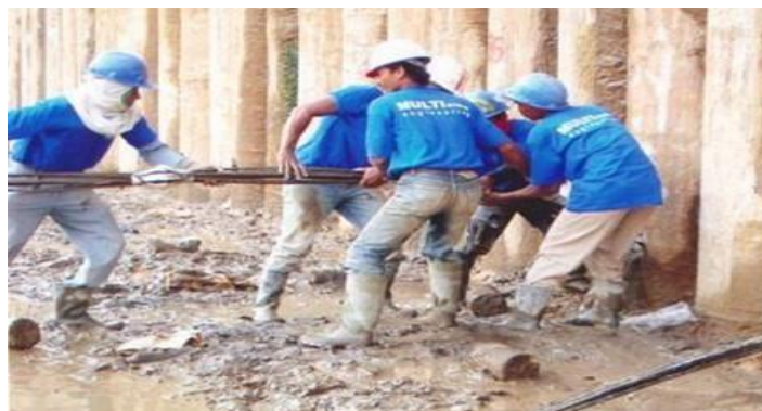
Gambar 4. 24 proses Install tali Anchor
