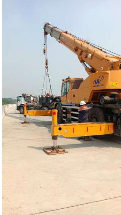
Gambar 2.3 Rough Terrain Crane
