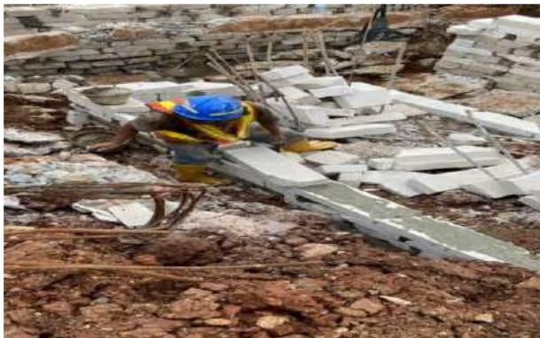
Gambar 4.16 Pemasangan bekisting tie beam
