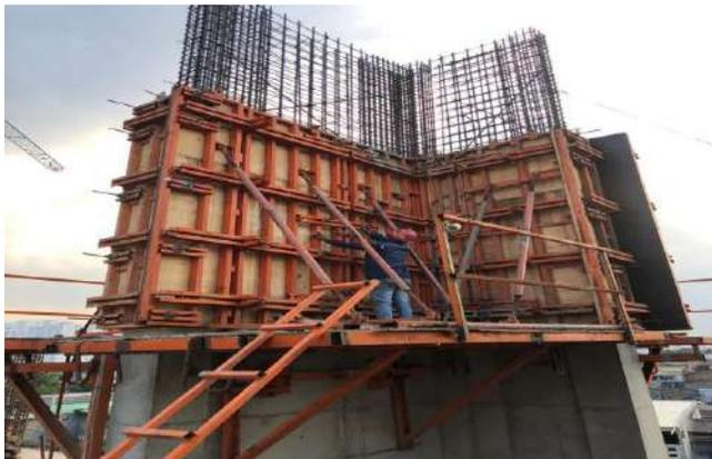
Gambar 4.32 Pemasangan bekisting *shear wall*
