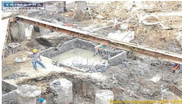
Gambar 4.10 *Bekisting pile cap*
