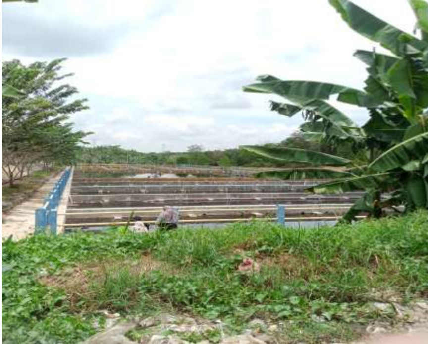
Figure 2.2 Lagoon System for Processing Leachate from Landfill
